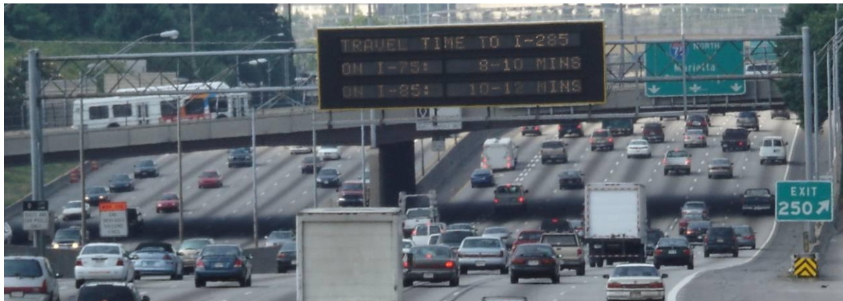
Figure 2.9. CMS on I-75/85 Northbound in Atlanta
