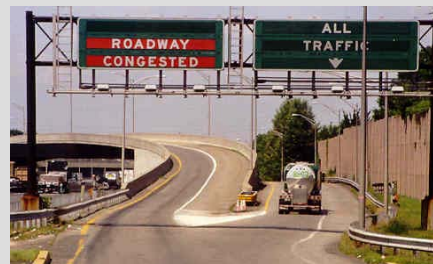
Figure 2. Entrance Ramp to the Dual-Dual Section of NJT
