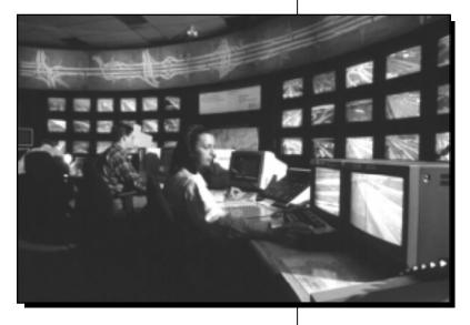
message signs. Variable message signs carry congestion management messages automatically. A separate system faxes traffic information automatically to an appropriate list of agencies and other organizations. Operators also have access to a Road Weather Information System monitor.
